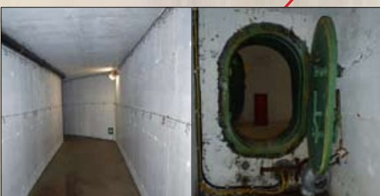
A commando headquarter has a size of 1500 m 2 (right) while a CuSy position uses less than 20 m 2 (left).
