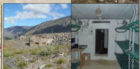
The Frøy defence line, built between 1981 and 1996, consists of 299 military complexes.
