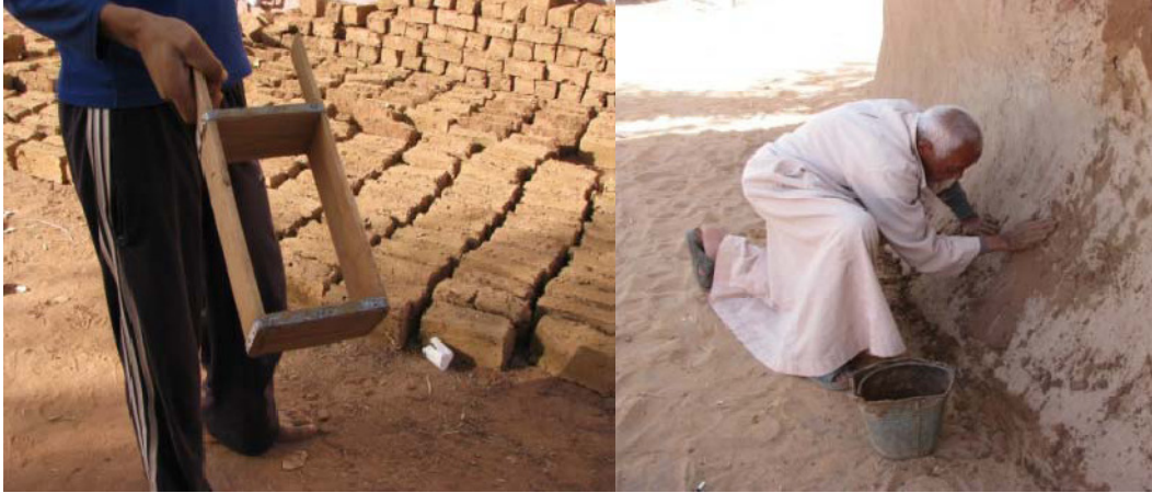
Fig:(3) Part of Building process :mud brick casting and plastering..
