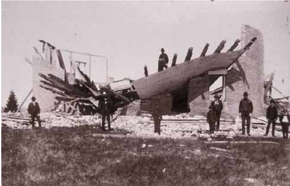
West Koshkonong Church, Dane County, Wisconsin, from 1852-1853 is well known from photographs. This photograph is taken after the rather unsuccessful attempt to demolish the church with the use of dynamite in 1893. It gives valuable information about construction details.
