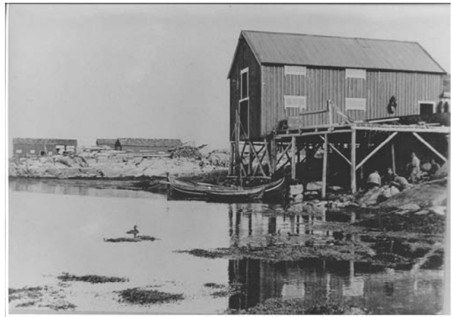
Figure 4. One of the old wharfs. In the background another wharf and boatsheds. Photo: 1912 Unknown. Property of Alf Sivertsen.
