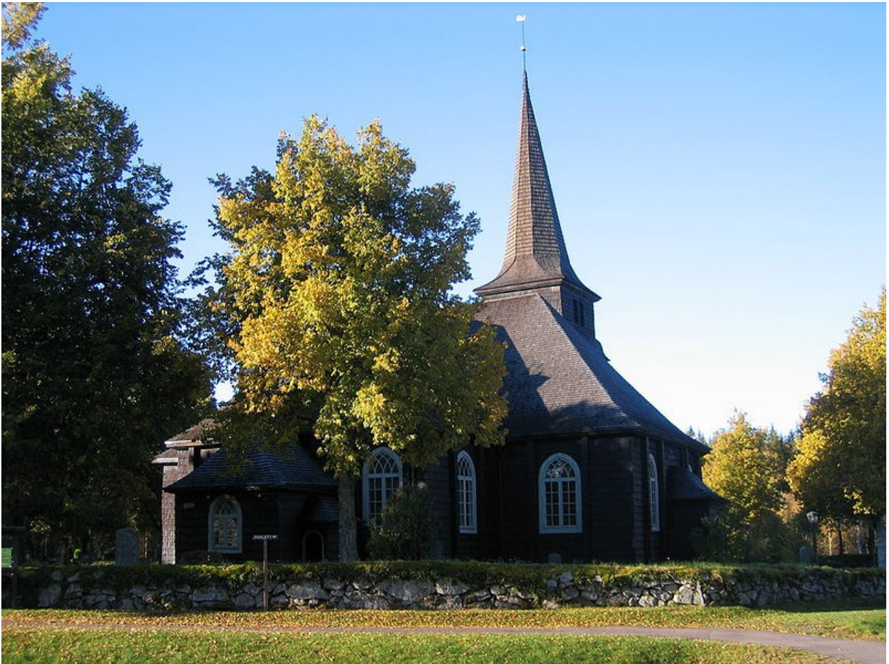
The object of the work: wooden cross church of Östmark (1765) covered by wooden shingles
