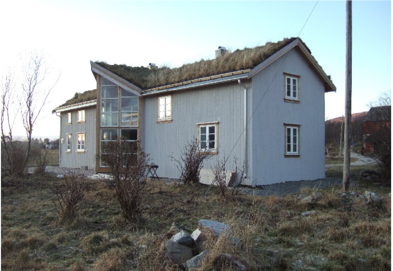
Saure farm, Steigen. Refurbishing a traditional farm building. Architect BOARCH arkitekter a.s./Gisle Jakhelln
