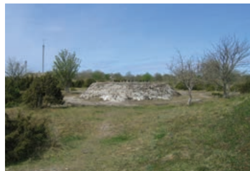
Concrete base with anchor bolts for 12-inch gun of Imperial Russian coastal battery. 1916. Sääre, Peninsula of Sõrve, Island of Saaremaa, Southwest Estonia. Photo: Kristel Valk, 2006
