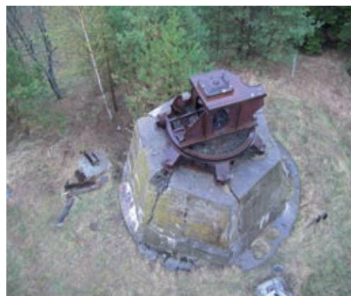
German station in the small island for Würzburg anti-aircraft radar, part of the Kamhuber Line. 1942. Island of Naissaar, North Estonia. Photo: Robert Treufeldt, 2011
