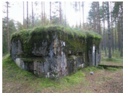
Observation bunker in the Estonian artillery proving ground. 1939. Kaber-neeme, Jõelähtme municipality, North Estonia. Photo: Robert Treueldt, 2010
