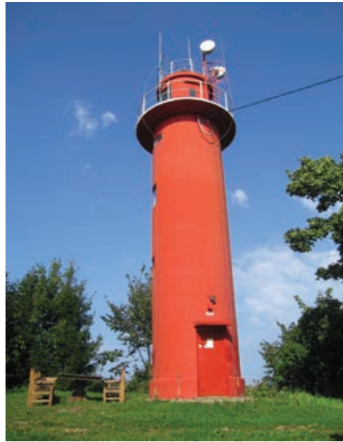
Built as a lighthouse, but during the wartime turned into the central fire control tower of Estonian coastal artillery. 1939. Lubja, Viimsi municipality, North Estonia. Photo: Robert Treufeldt, 2013
