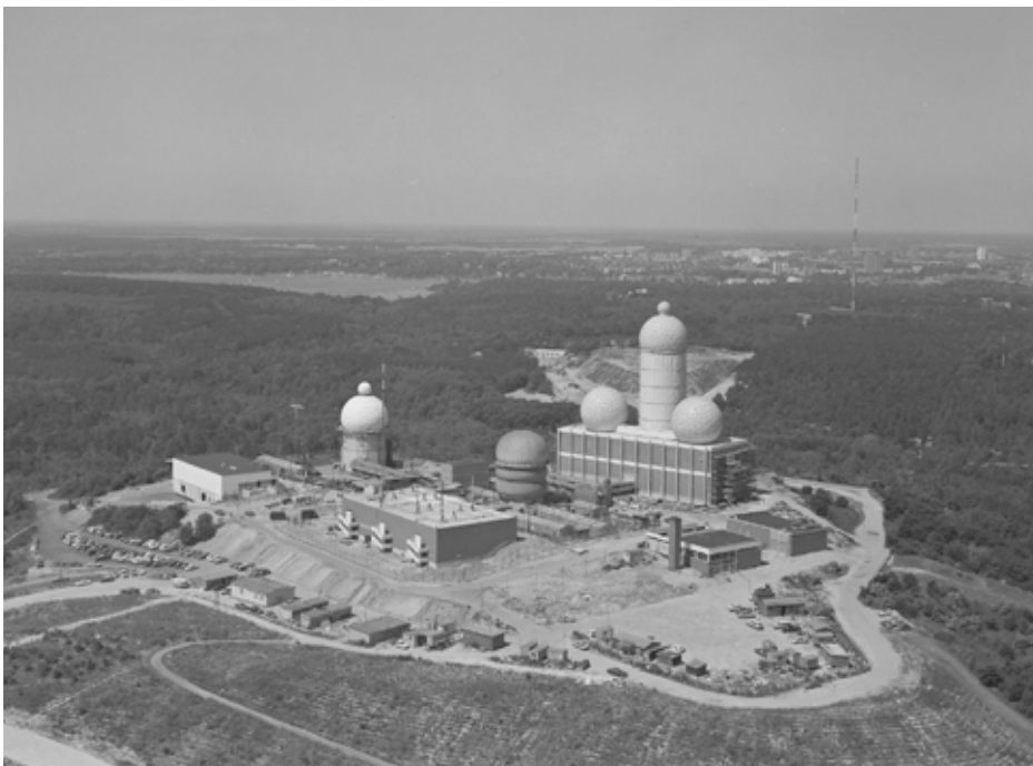
US National Security Agency listening station on the top of Teufelsberg, a man-made hill, Berlin, 1971
