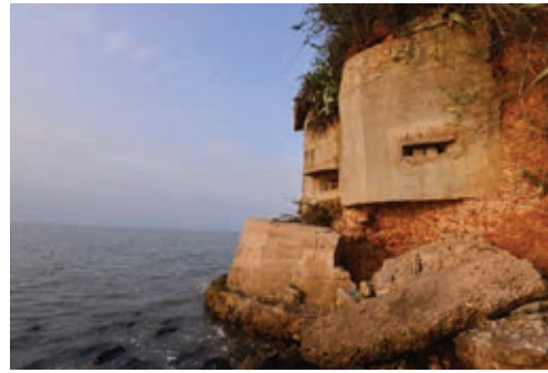
Barracks were demolished so as to return the land for the civilians
